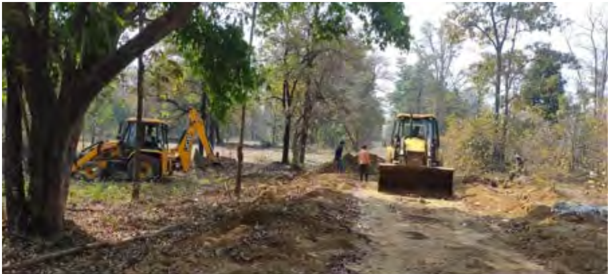
Figure 22: Road construction near Chilparas
