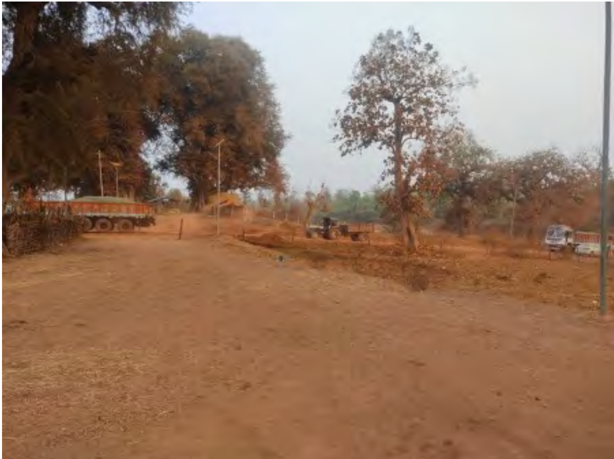
Figure 30: Chhotedongar: dust and potholes
