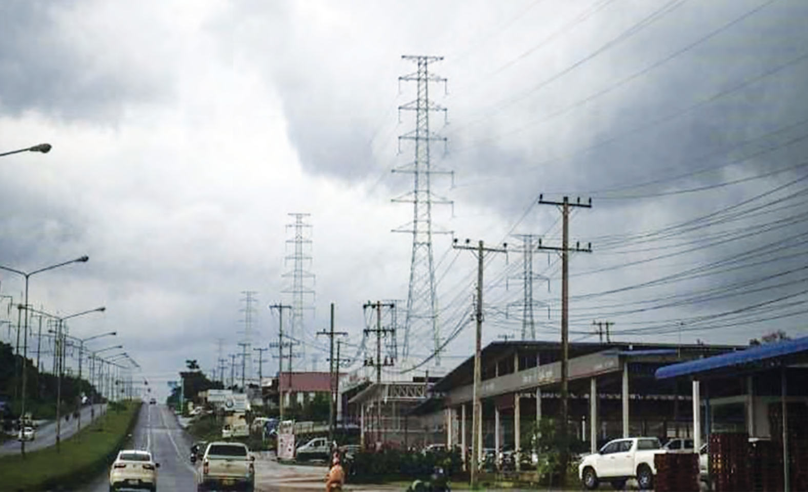
• New pylon towers used in power distribution, coming from hydro power plants, run through Pak Se District in the Champasak Province of Laos on July 25, 2018 (Phys Org, 2018).
